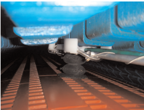
Air bladder holding the carriage in place while the glue cures. The rotor is at the bottom of the photo.
